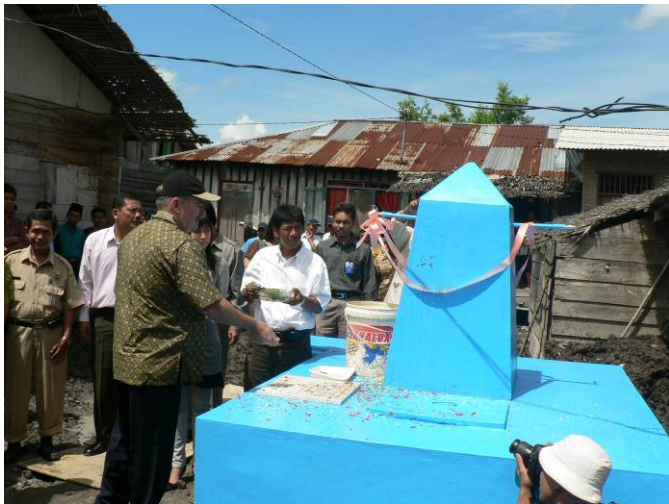
Russ Dilts ESP Advisor “teping tawar” the Reservoir with capacity 4 m3 to serve over 150 households
